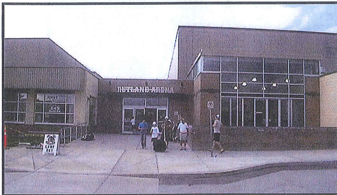
4. East entrance, Rutland Arena.
